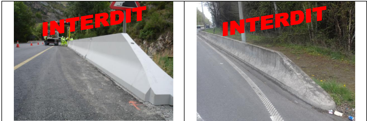
Figure 39 – Enfouissements interdits.
